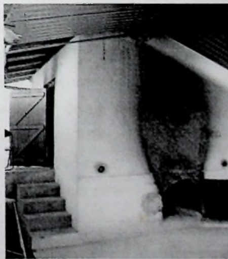
Fig 5: Conventional type Smoke House
