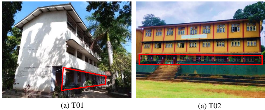
Figure 7-4. Open Ground Storey of T01 and T02 buildings
