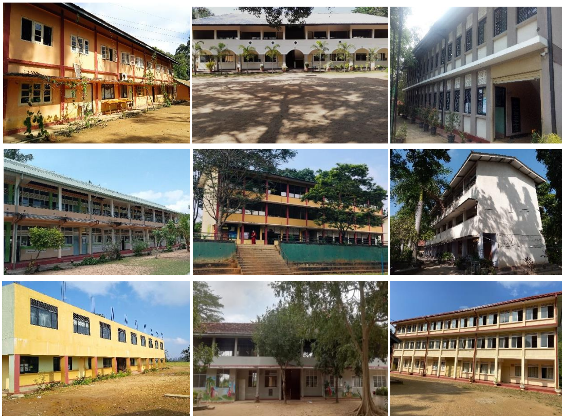
Figure 4-2. Some of the surveyed school buildings (two and three storeys)
