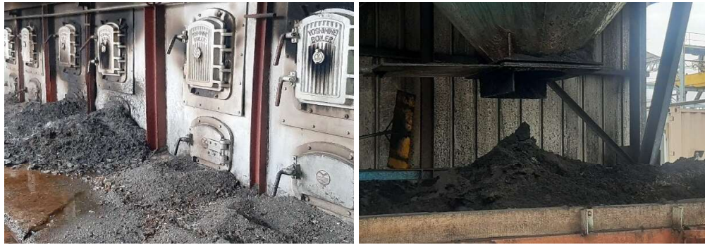
(a) Bottom ash-collected from the bottom of the boiler (b) Top ash - collected from electrostatic separators
