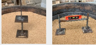
Two prototype footings
