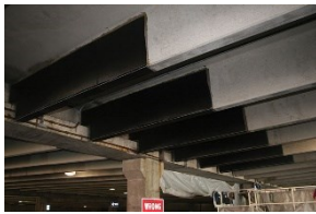
FRP-Strengthened Concrete Beams
