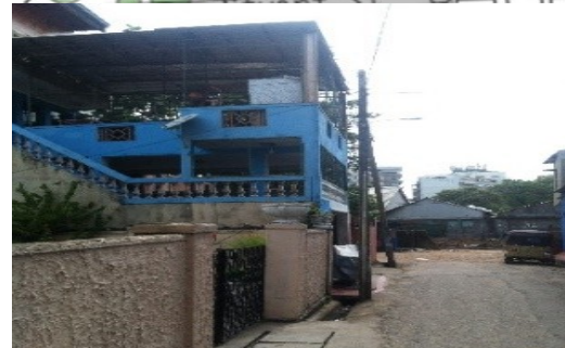
Fig 43: View of end space from Church Street Source: Compiled and captured by Author
