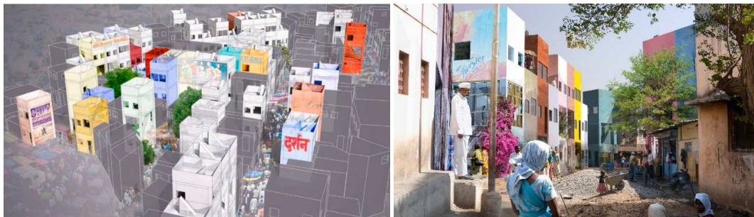
Fig.2: New archipelago of incremented kaccha houses rising from a context of well-built permanent homes in a typical slum- Pune, India Source: www.archdaily.com
