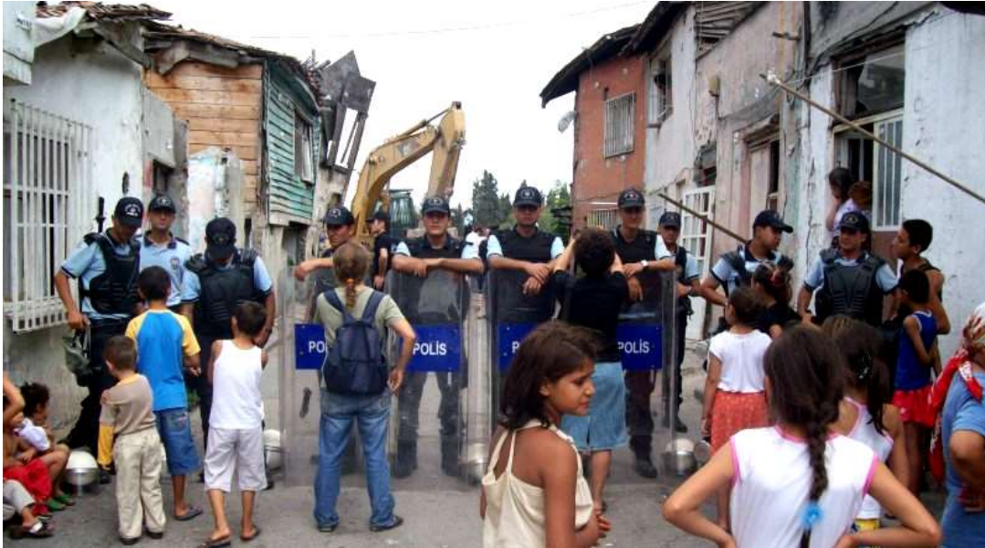
Fig. 12: Demolishing day in the neighbourhood, 2008 Source: http://sulukulegunlugu.blogspot.com/
