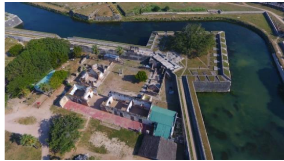
Figure 12- Aerial view of the Gelderland Bastion and Queen's House - Jaffna Fort (Source: Author)
