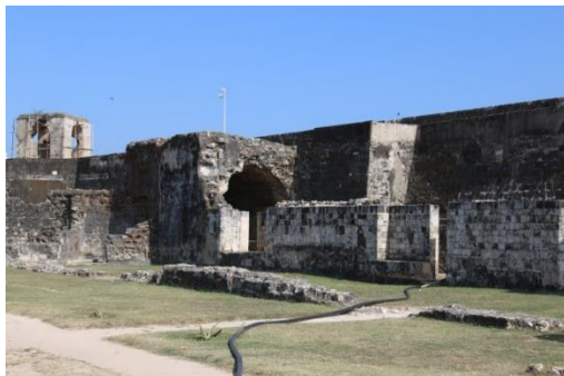
Figure 13- Remains of the guard rooms - Jaffna Fort (Source: Author)
