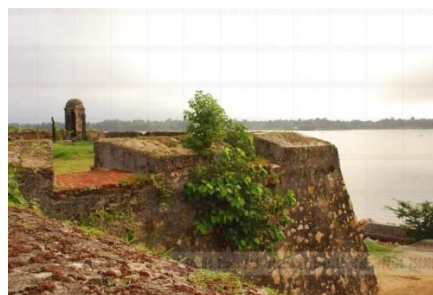
Figure 17- Building A, shows similar features to the Colombo Dutch Hospital (Studio Times Pvt Ltd)
