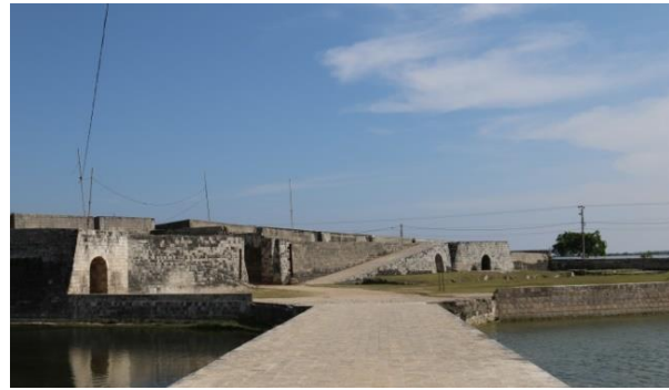
Figure 10- Internal view of the outer circuit south ravelin from the entrance gate - 2019 - Jaffna Star Fort (Source: Author)
