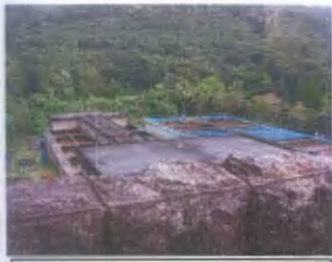
Labugama Treatment Plant
