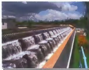
Ambalate Treatment plant
