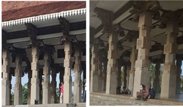
Figure 12: PPPT activities near columns at Independence square - columns Source: Author
