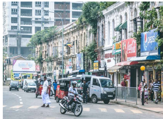
Figure 10 : Shop houses marked for demolition in Slave Island Source: (roar.media, n.d.)
