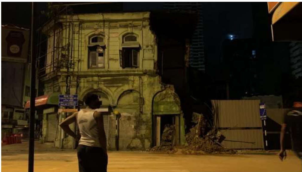
Figure 8 : Collapse of the De Soysa Building (Thomas, 2021a)
