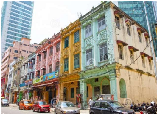
Figure 9 : Shop houses renovated in Kuala Lumpur Source: (www.dreamstime.com, 2013)
