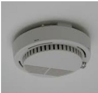
Figure 24: Smoke detector
