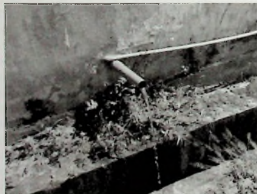
Figure 13: Grey water draining directly into the canal
