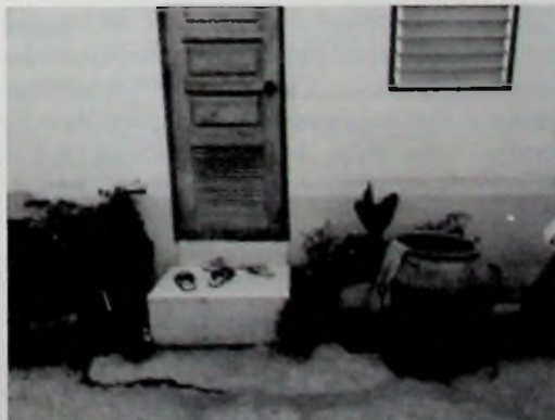
Figure 7: Flood line on Bang Bua homes from 2011 floods
