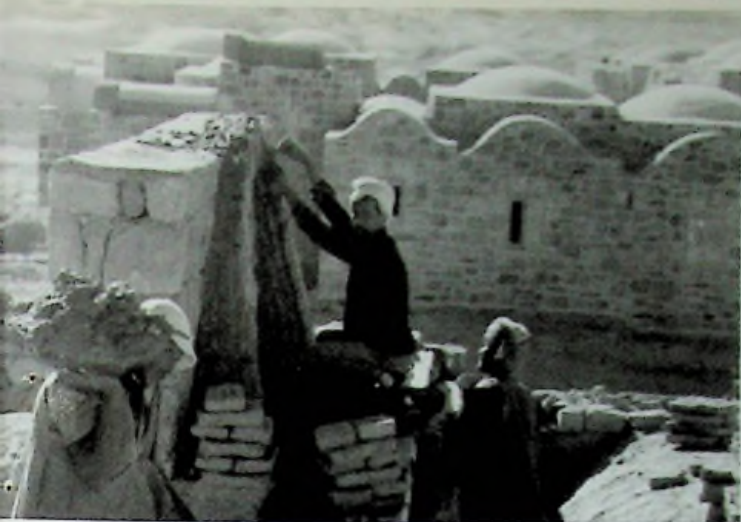
Figure 10: Building a Nubian Vault in al Quseir
