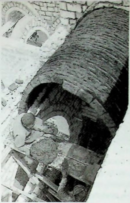
Figure 3: Building a Nubian Vault
