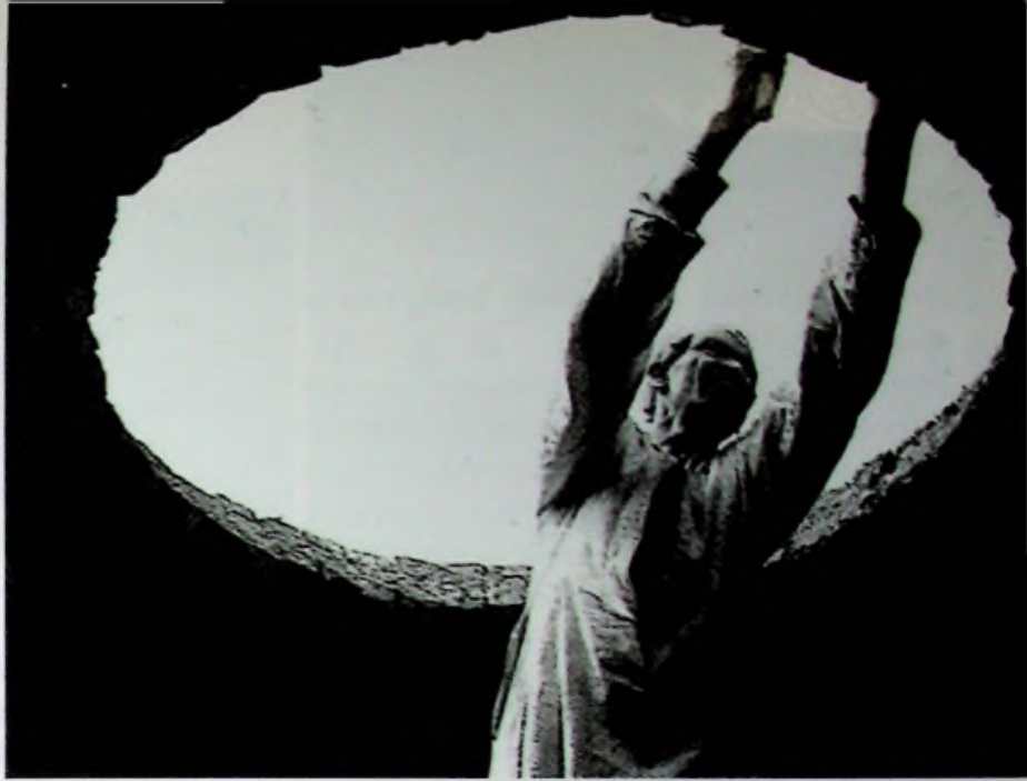
Figure 4: Building a dome
