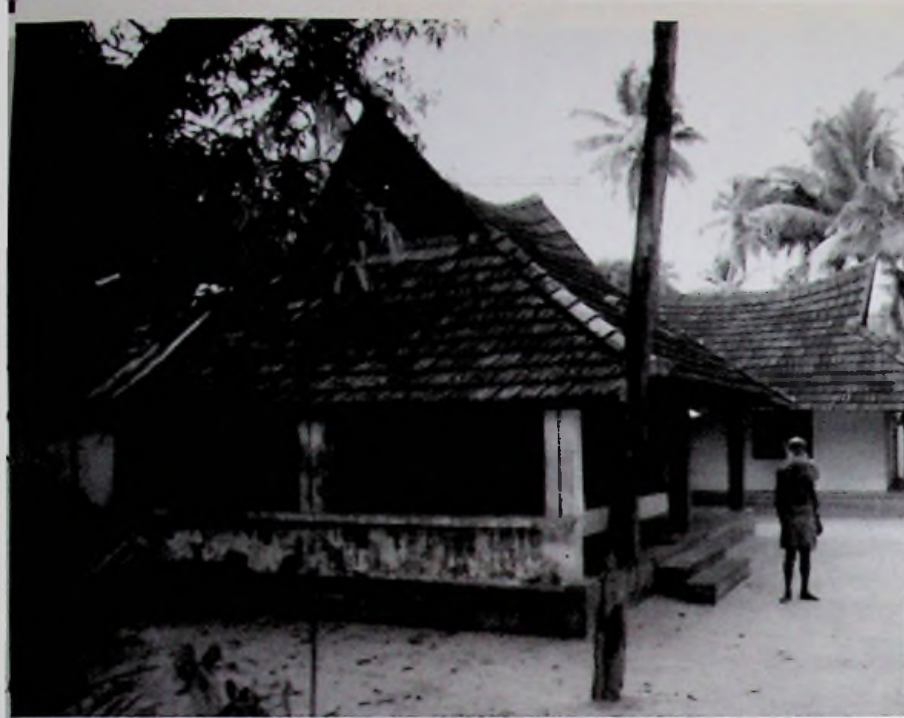
Figure 4: A single aroodam house with pathayappura, at chavara, Kulangara house, chavara, kollam, kerala .the koodu is supported by the aroodam(wall plate supported by the wall and the wooden pillars.
