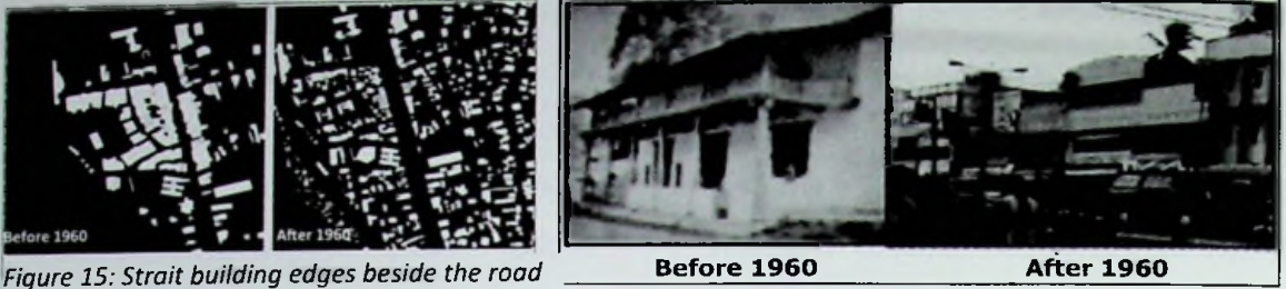
Figure 15: Strait building edges beside the road
