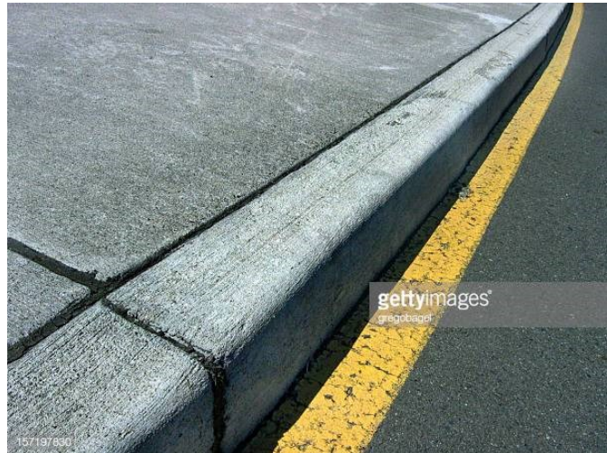
Figure 2.3: Image of curb (source: gettyimages)
