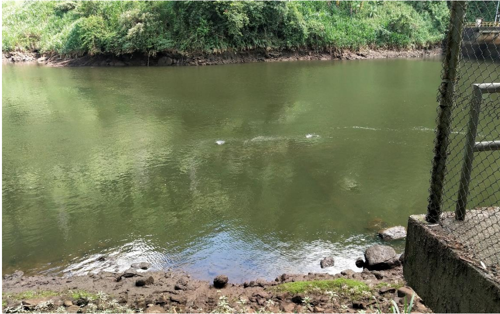
Figure 1- 3: Free surface vortex at Samanala Hydro Power Intake
