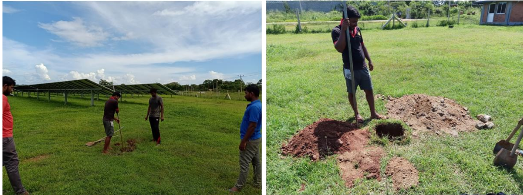
Figure 6.15: Borehole excavation
