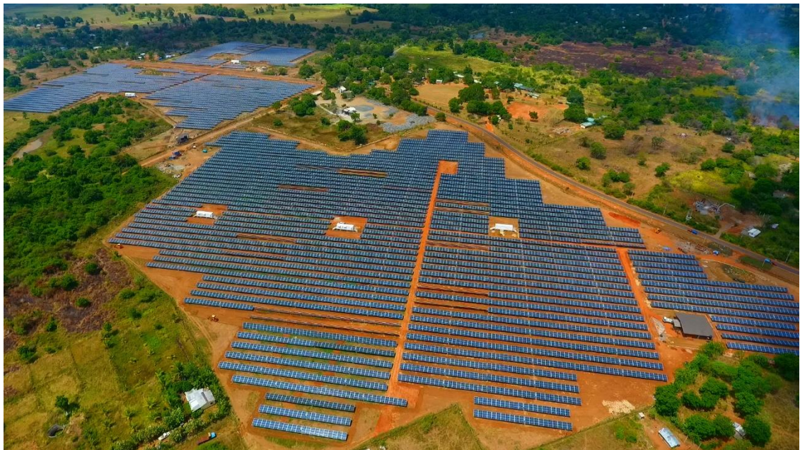
Figure 5.6: Selected area for the field measurement – Location 1
