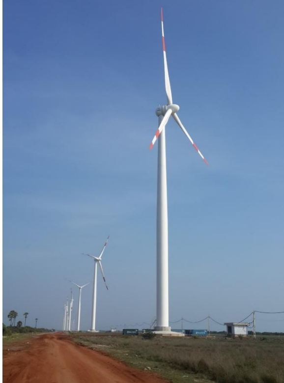
Figure 5.15: Selected area for the field measurement – Location 2
