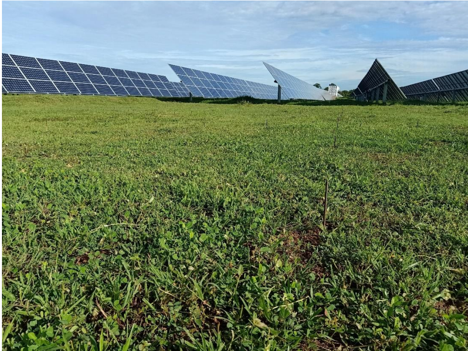
Figure 5.10: Earth Resistivity probe arrangement – Location 1
