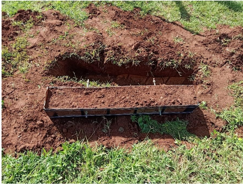
Figure 5.11: Topsoil excavation and soil box filling
