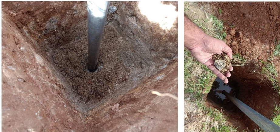
Figure 6.20: Borehole up to 3.5 m
