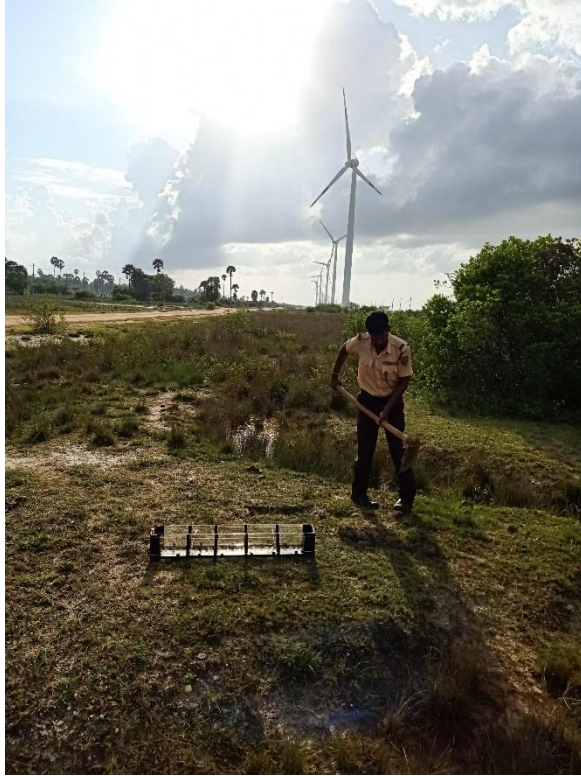
Figure 5.19: Top soil excavation and soil box filling
