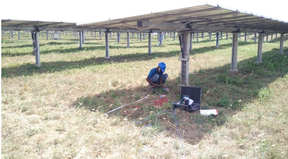
Figure 5.8: Earth Resistivity Measurement
