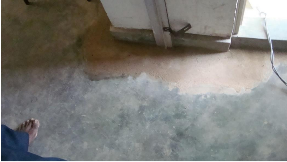
Figure 4-8: Remedial action taken on Goda Canteen rooftop - 1
