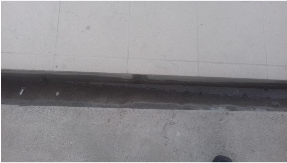
Figure 4-56: Rooftop drains into which water gets drained beneath the tile surface - 2
