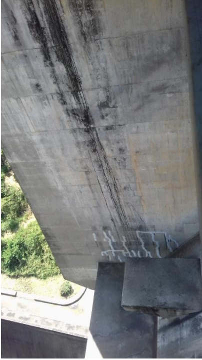
Figure 4-63: Affected surfaces were injected with waterproofing solutions - 1
