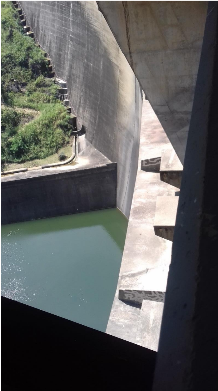
Figure 4-64: Affected surfaces were injected with waterproofing solutions - 2
