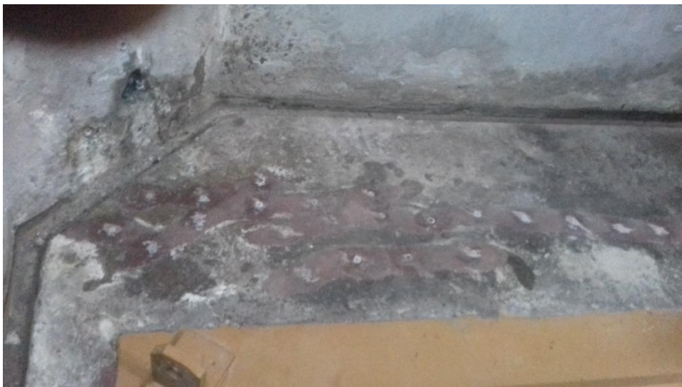
Figure 4-70: Surface injected with waterproofing solutions - 2
