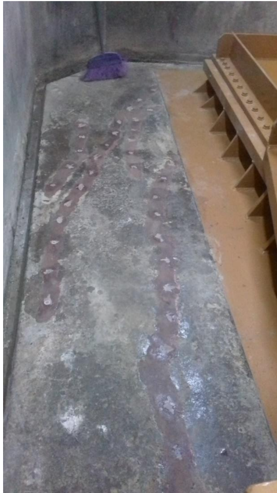
Figure 4-69: Surface injected with waterproofing solutions - 1
