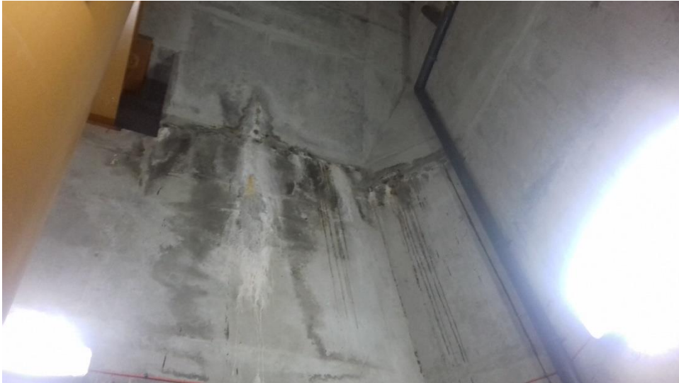
Figure 4-72: Surface injected with waterproofing solution from top level - 2
