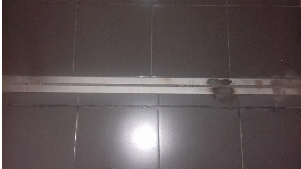
Figure 4-45: Construction joint line in floor level of 7 th floor
