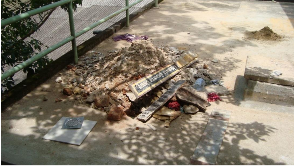
Figure 4-10: Remedial action taken to prevent water leakage
