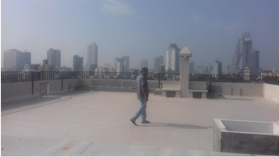
Figure 4-59: Post application of waterproofing solution at rooftop level
