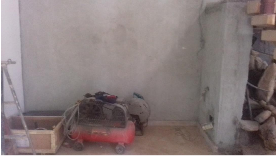
Figure 4-25: After application of cover plaster - 1
