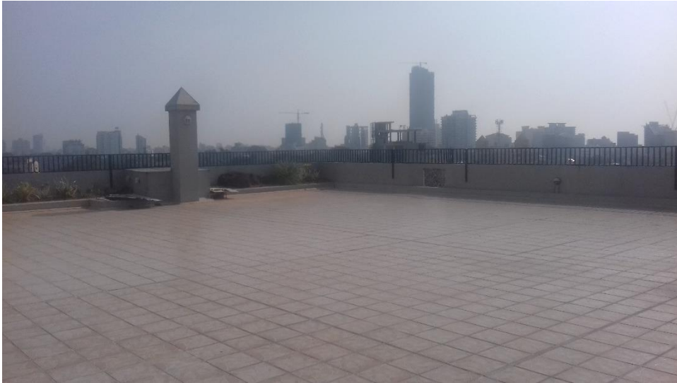
Figure 4-58: Rooftop surface to be finished
