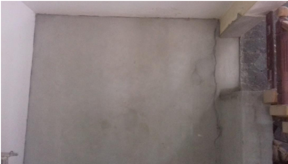
Figure 4-26: After application of cover plaster - 2
