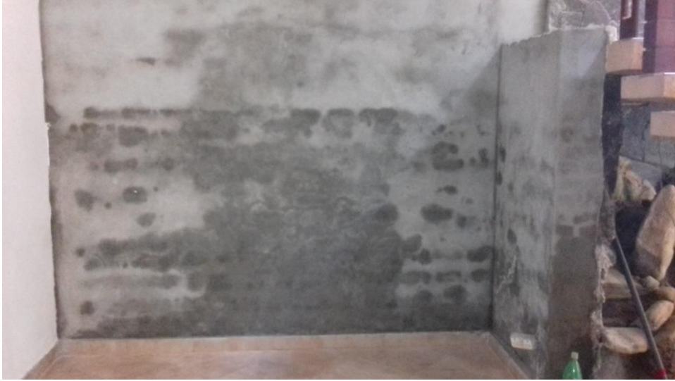
Figure 4-23: After surface preparation for waterproofing
