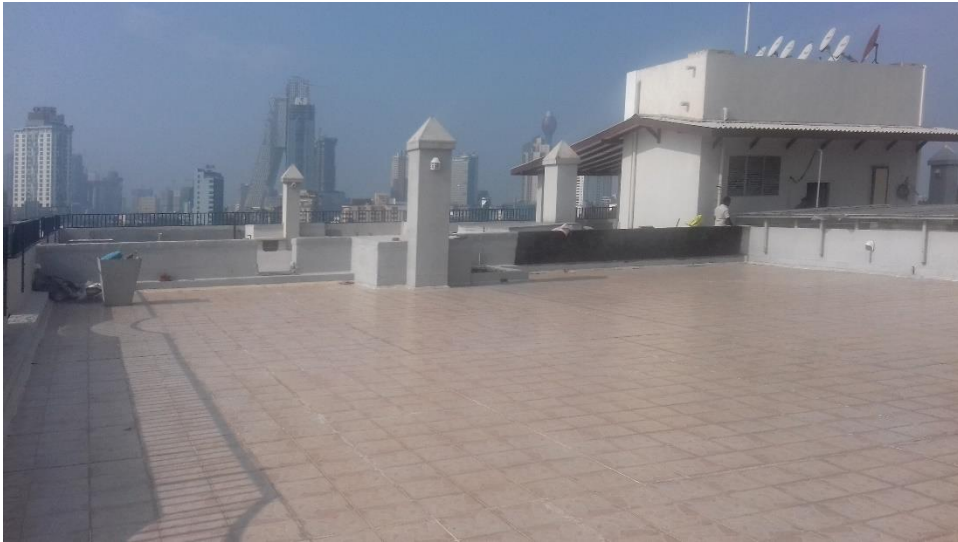
Figure 4-60: Finished surface and unfinished construction joint line of rooftop
