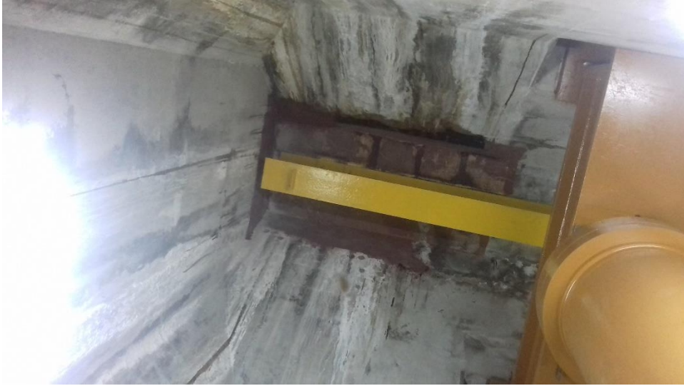
Figure 4-71: Surface injected with waterproofing solution from top level - 1
