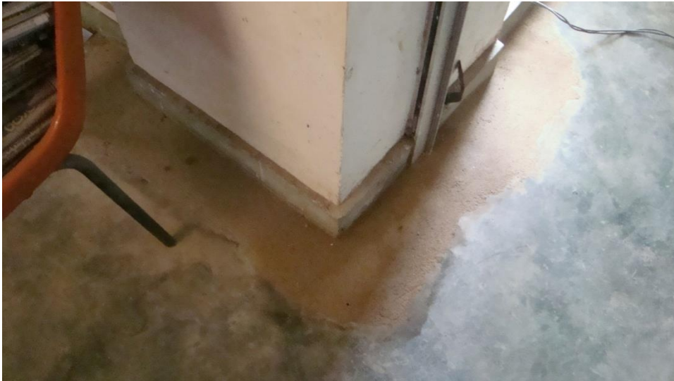
Figure 4-9: Remedial action taken on Goda Canteen rooftop - 2
