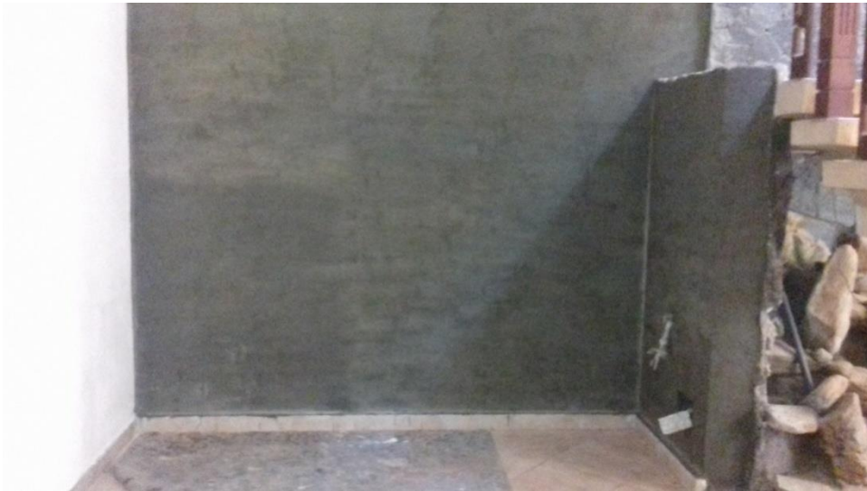
Figure 4-24: After application of waterproofing
