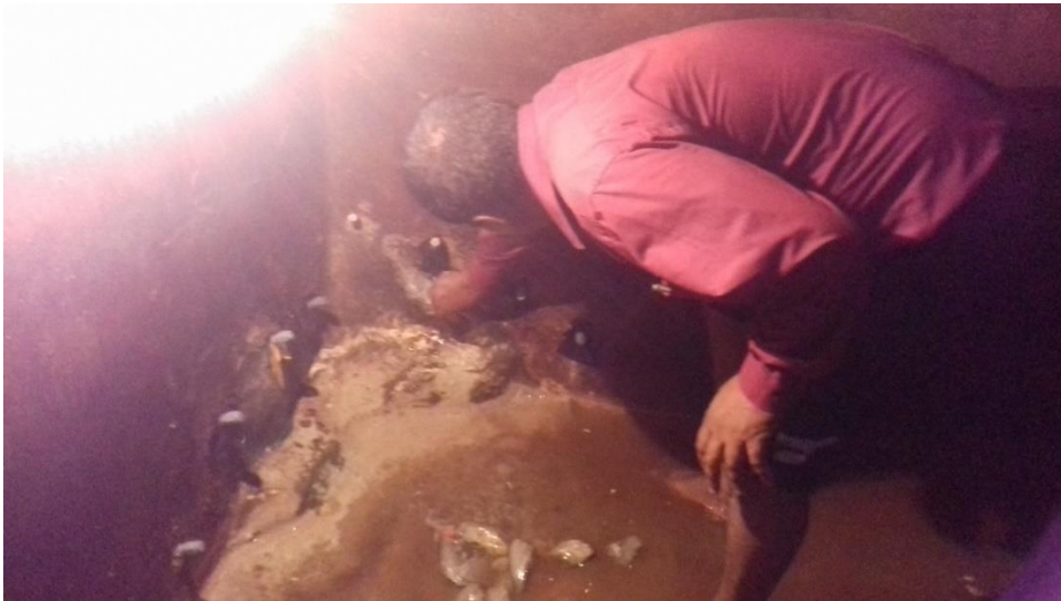
Figure 4-39: Non-return nozzles fixed to inside walls for the injection process - 2
