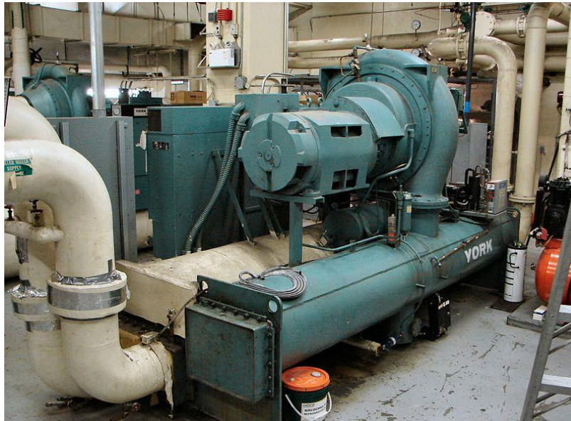
Figure 5 : Chiller Plant [4]
