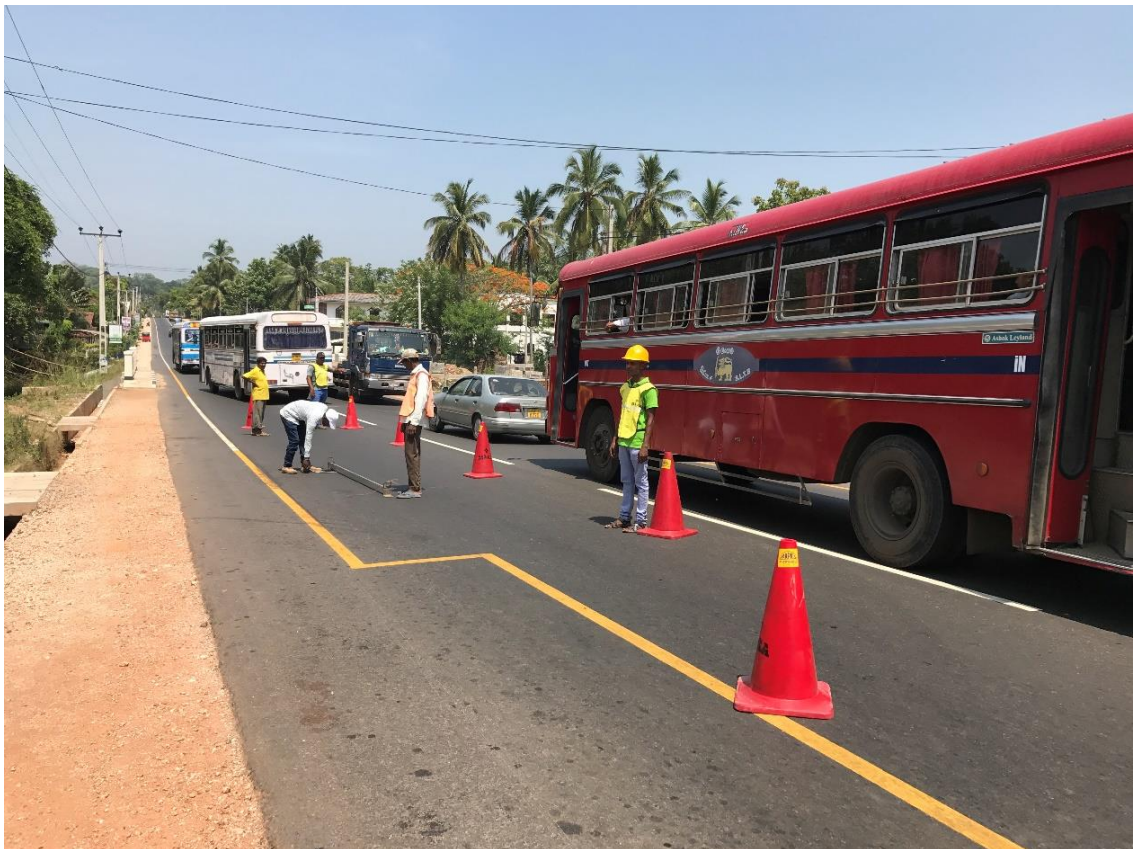
Figure 3.8 Survey for longitudinal surface regularity in corrugated section (40+200 km)
