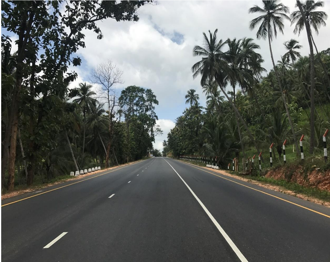
Figure 3.5 Upward view of non-corrugated pavement section (67+700 km)
