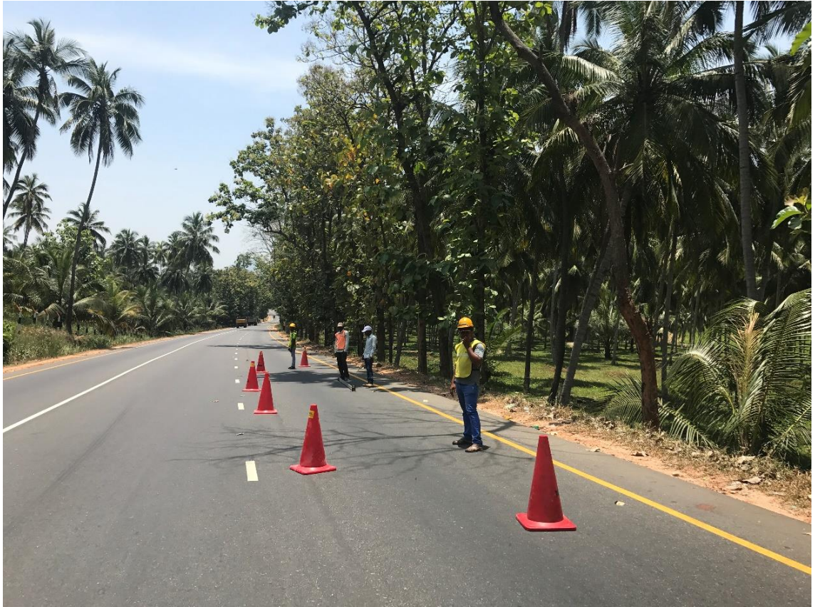
Figure 3.9 Survey for longitudinal surface regularity variations in non-corrugated section (60+400 km)
