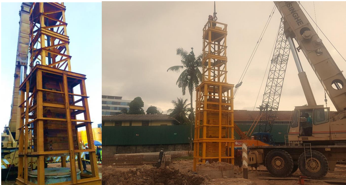
Figure 16. HSDLT arrangement with guide frame and 28 ton drop hammer.
