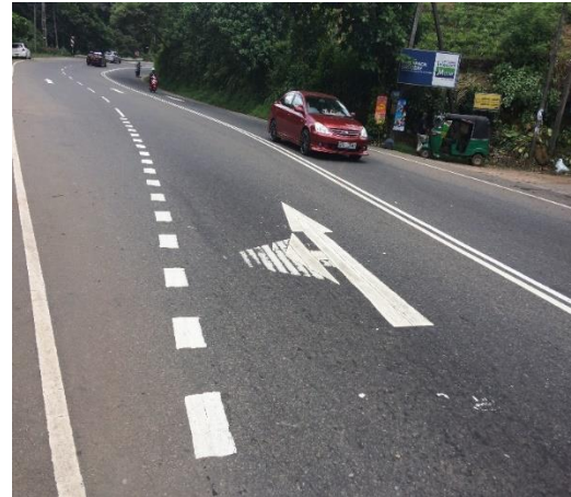
Figure 3.5 Climbing lane upstream point
