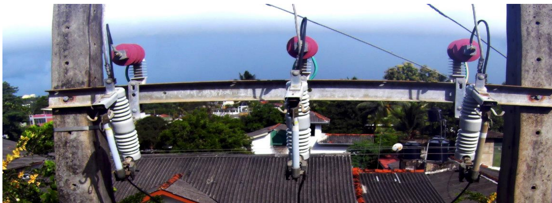
Figure a : DDLO assembly
