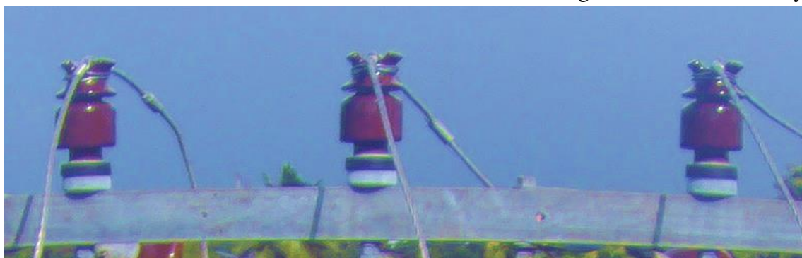
Figure b : Insulation assembly
