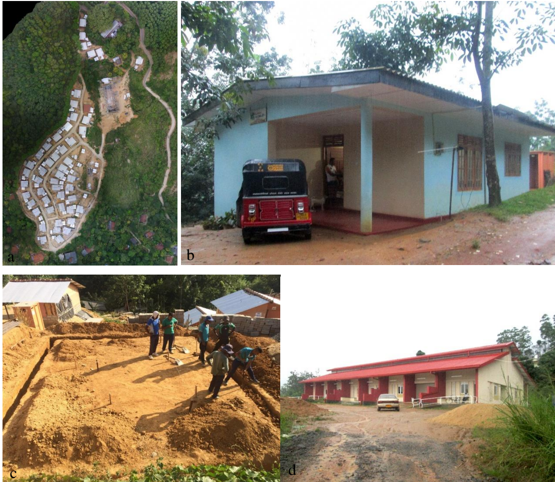
Figure 3-6: a) relocated site of Case B, b) completed house. c) ongoing construction of case B. c) completed community center of case B Source: a and c images- NBRO
