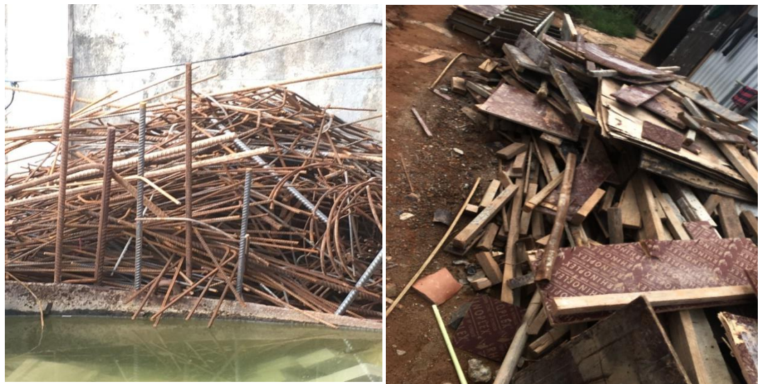
Figure 4.3 : Steel and wood waste collection in Case C
