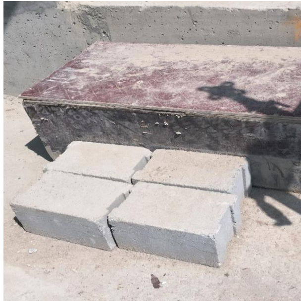
Figure 4.11 : Concrete cubes used for temporary works in the Case F
