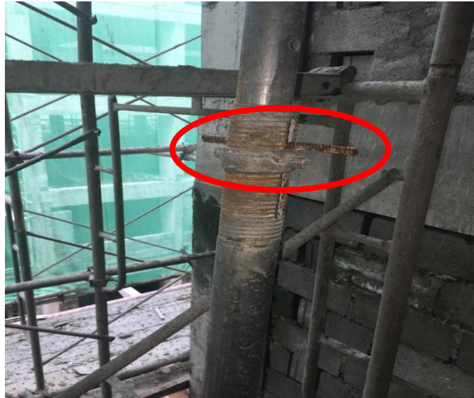
Figure 4.9: Steel offcuts used in acro jacks in Case E
