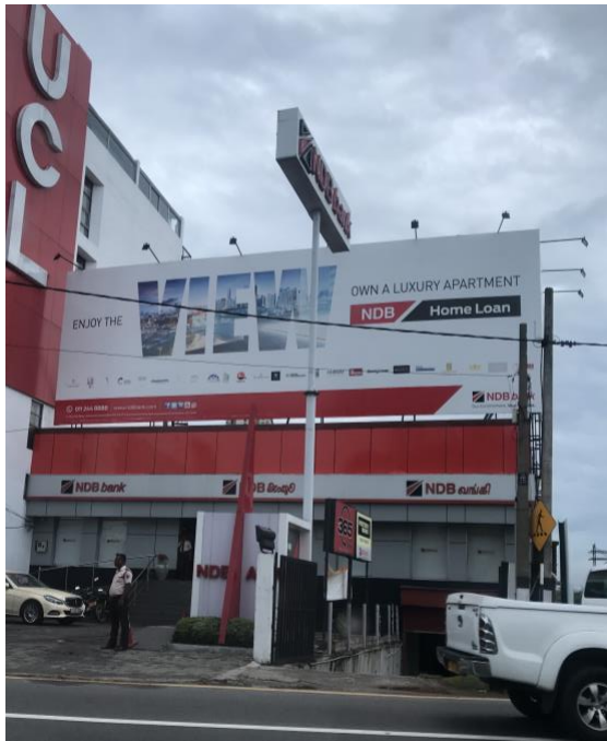
Figure 30: The Bank exterior
