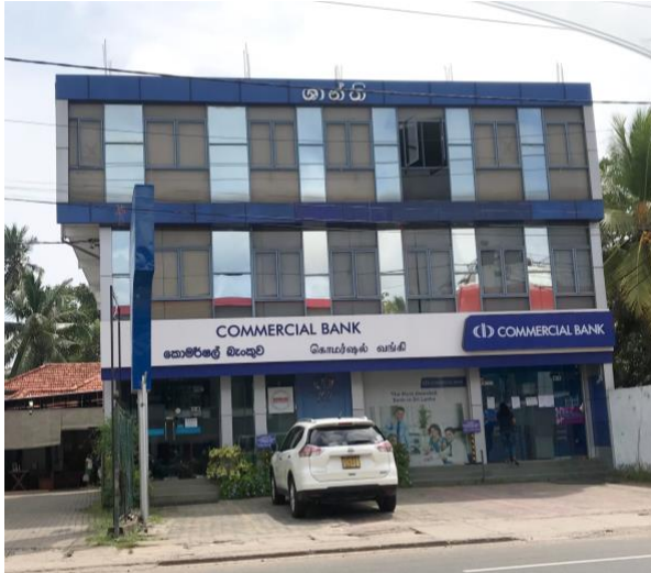
Figure 54: The Bank exterior
