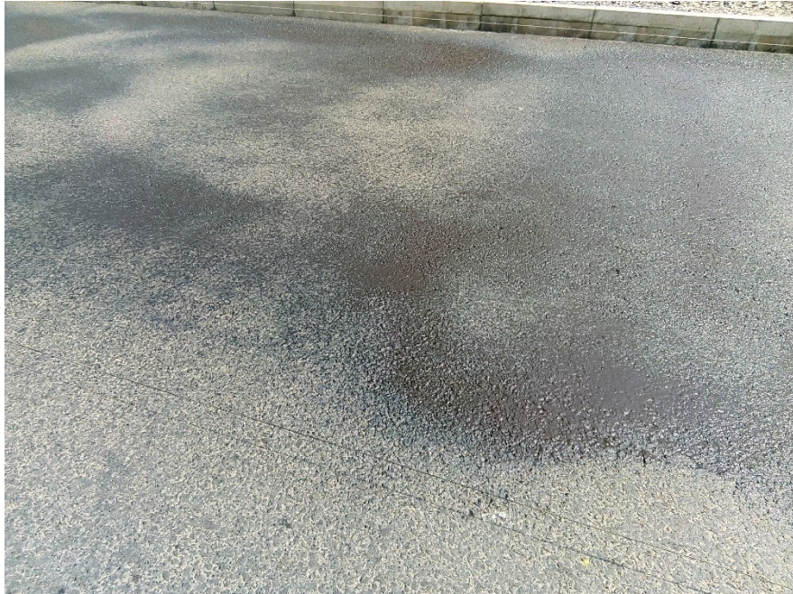
Figure 12. Tacked surface of manual application
