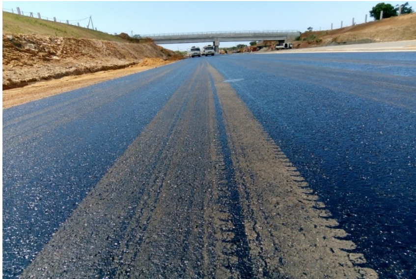
Figure 2. Tack coat picked up by haul truck
