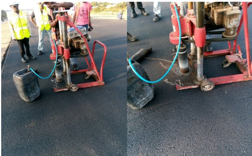
Figure 23. Coring process
