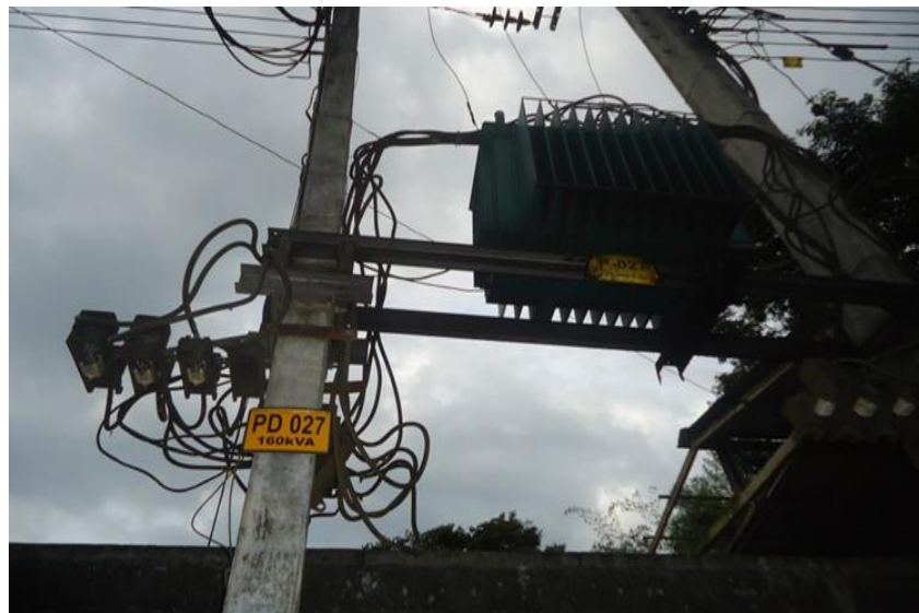
Figure 7: Poor workmanship
