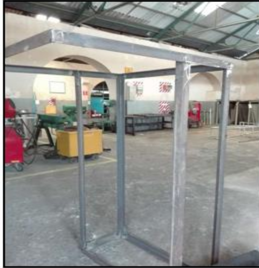
Figure 4.3: Fabrication of the Supporting Structure
