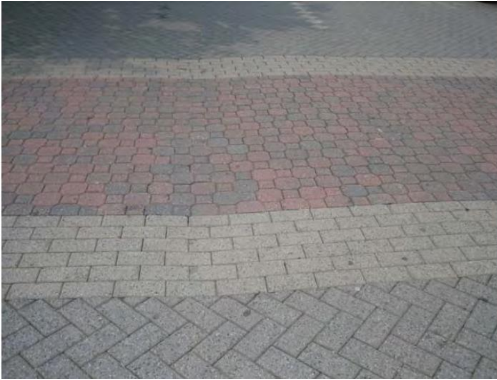
Figure 3-6 Sample distress (Medium severity)
