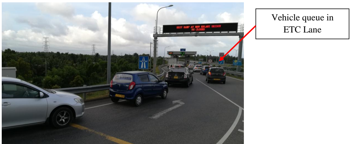
Figure 9: Developing of vehicle queue in Entrance toll plaza -D at Ja Ela IC
