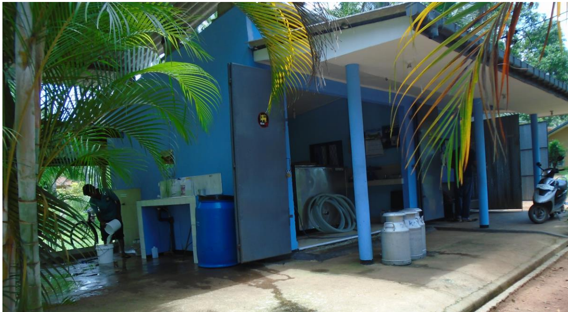
Figure 2.7.2: A typical milk chilling center of a large scale dairy manufacturer
