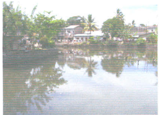
Fig : (40) Kirulapone canal divided in to two parts As Wallewatta canal and Dehiwala out let From the end point of Thalakotuwa garden.
