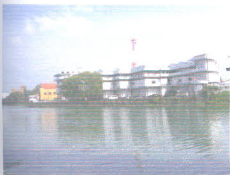
Figs :( 85) Akbar Telecom building
