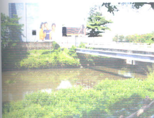
Fig : ( 32 ) View of the Duplication road, newly constructed bridge.
