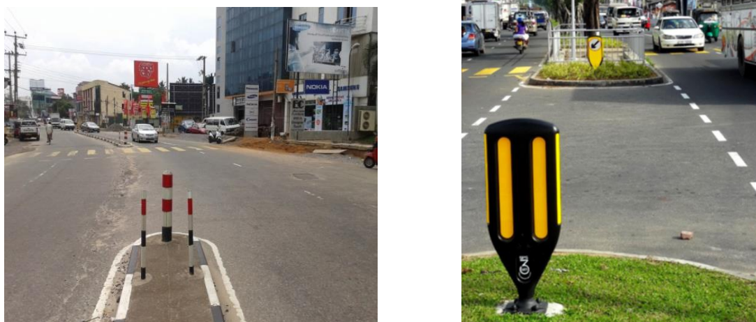
Figure 1-1 Existing Median Openings
