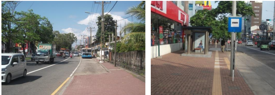
Figure 4.3.3.1. Bus bays at Moratuwa (left) and Kollupitiya (right) at Galle road
