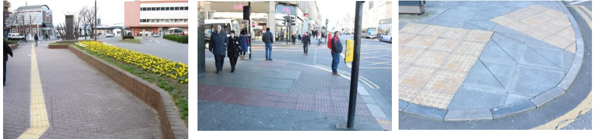
Plate 4.4.2.1: Tactile pavings observed in Kyushu (left), Japan and Aberdeen, UK (middle and right).
