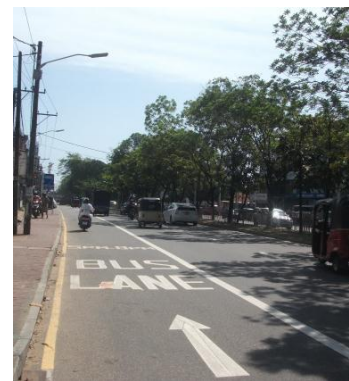
Plate 4.3.4.2: Road Markings at the Galle road
