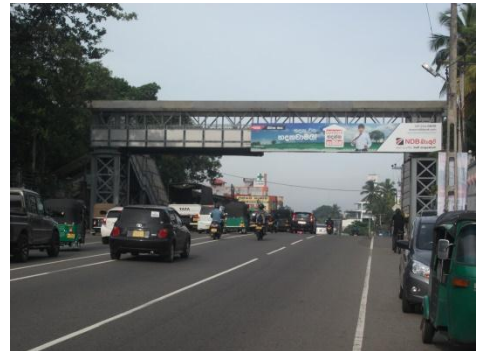
Plate 4.3.1.6: Pedestrian overpass at Pannipitiya
