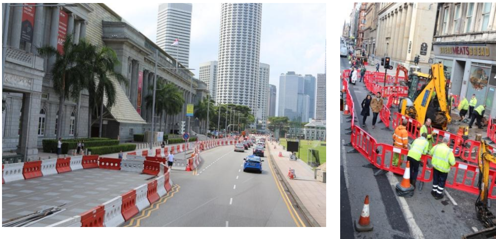
Plate 4.4.20.1: Barricaded construction areas in Singapore.
