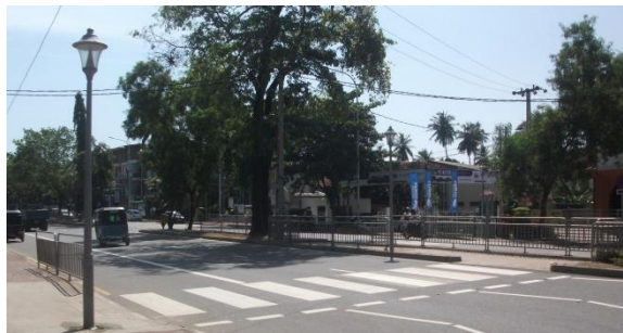
Plate 4.3.1.3 a: A Zebra crossing at Galle Road, Moratuwa with beacon lights
