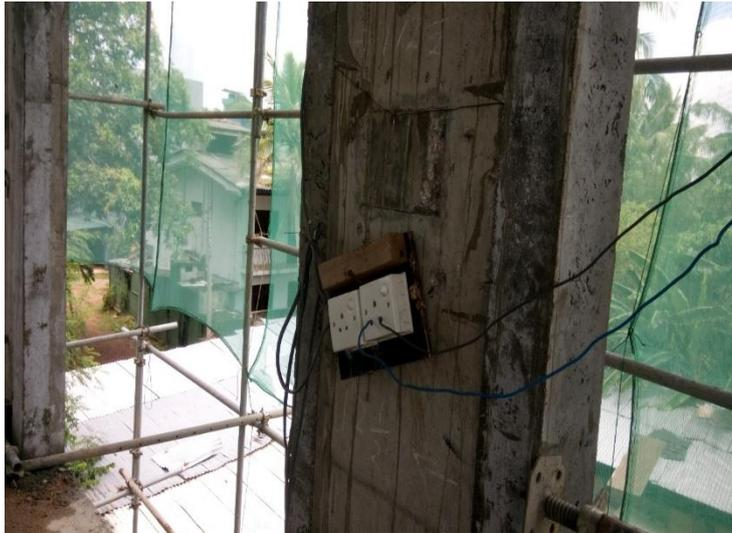
Figure 7.6 unsafe conditions in construction sites
