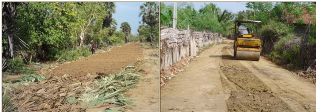
Figure 1.1: A traditional method of road construction in Northern Province
