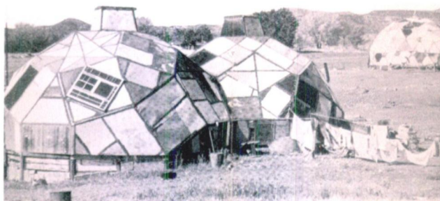
Fig. 27 Drop city, Colorado, built of panels cut from the roofs of scrapped cars and vans.
