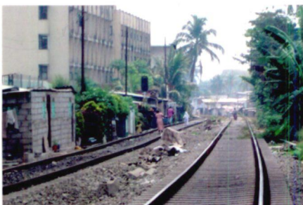
Plate – 3.17 Buildings closed to the rail way line
