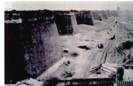
Plate -1.10 The wall of Beijing base is 16 ft wide, their breadth at the top about 40 ft, their height also averages 40 ft.
