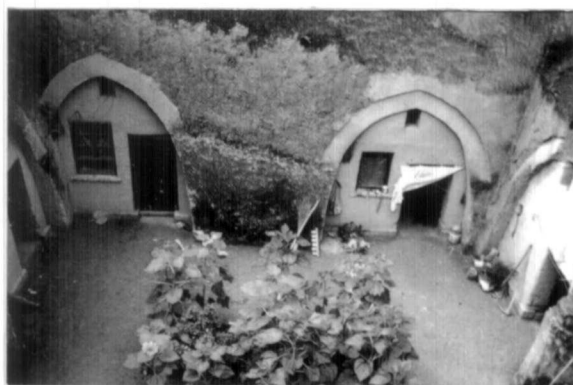
Image 2.2 : Underground Cave Houses in China. These houses are a very effective way of living. Keeps houses warm during the night and cooler during the day.
