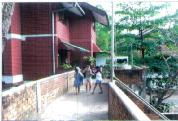
Image 3.37 : the walkways and the space in front of the entrances which are personalized with plants.
