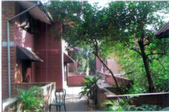
Image 3.36 : showing how the buildings were designed without harming the trees on site.
