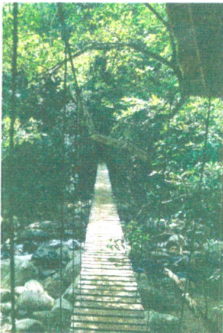
Figure 41 Bridge through Kirindi Oya
