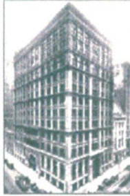
Fig. 1.3 First steel skyscraper: Home Insurance Building
