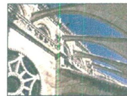
Fig. 1.2 Flying buttresses: Notre Dame Cathedral
