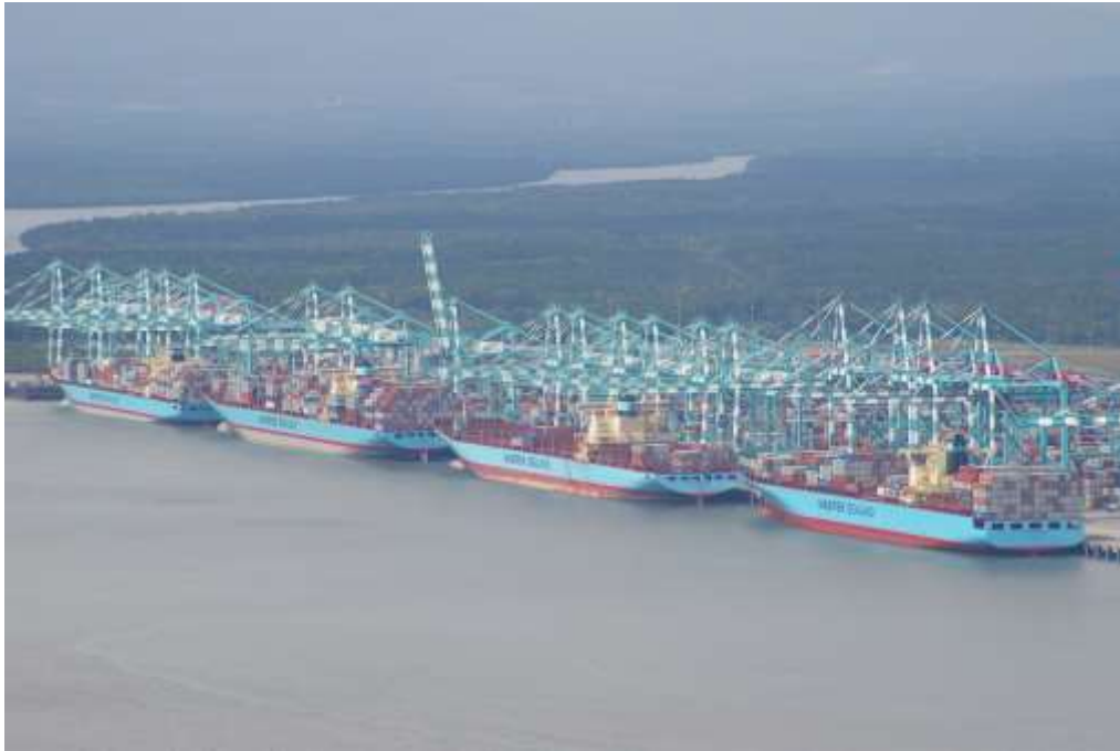
Figure 2.15-2: Continuous berthing layouts- Port of Tanjung Pelepas, Malaysia
