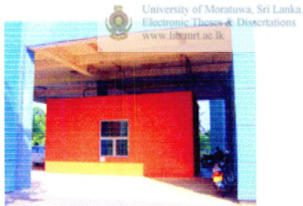
Figure 96 : Red box at the car park
