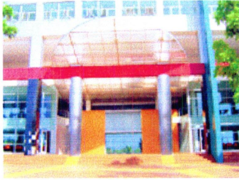
Figure 93 : Red beam of the main entrance creates a barrier.
