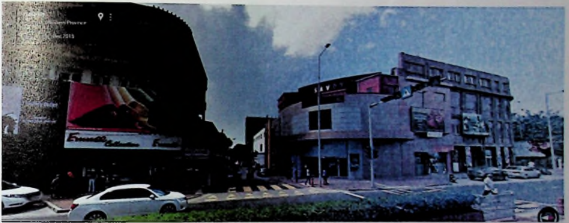
Figure 43: Savoy Building today
