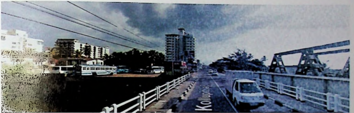
Figure 27: Exit at Marine Drive
