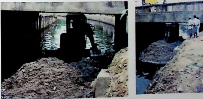
Figure 82: Dredging work at the Kirulapone canal
