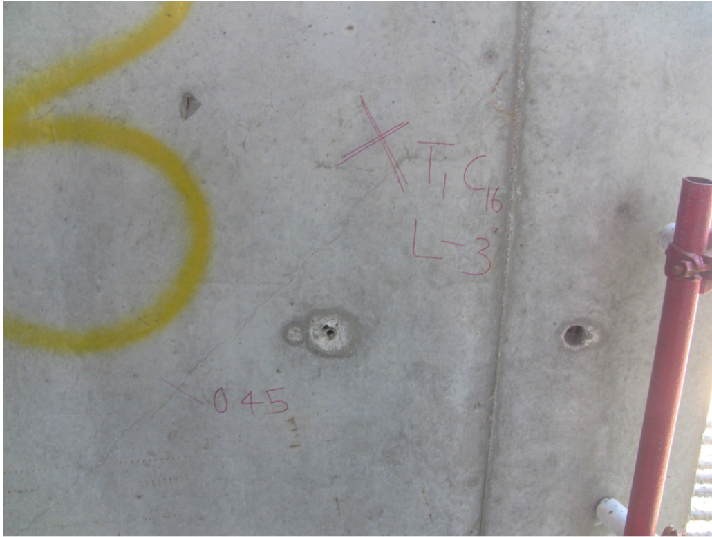
Figure 12: Diagonal crack observed [Project in Colombo]
