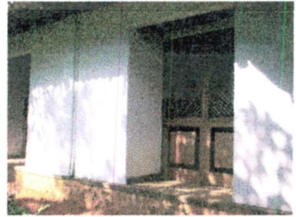
Figure3. :lighting of the trees taken to the building
