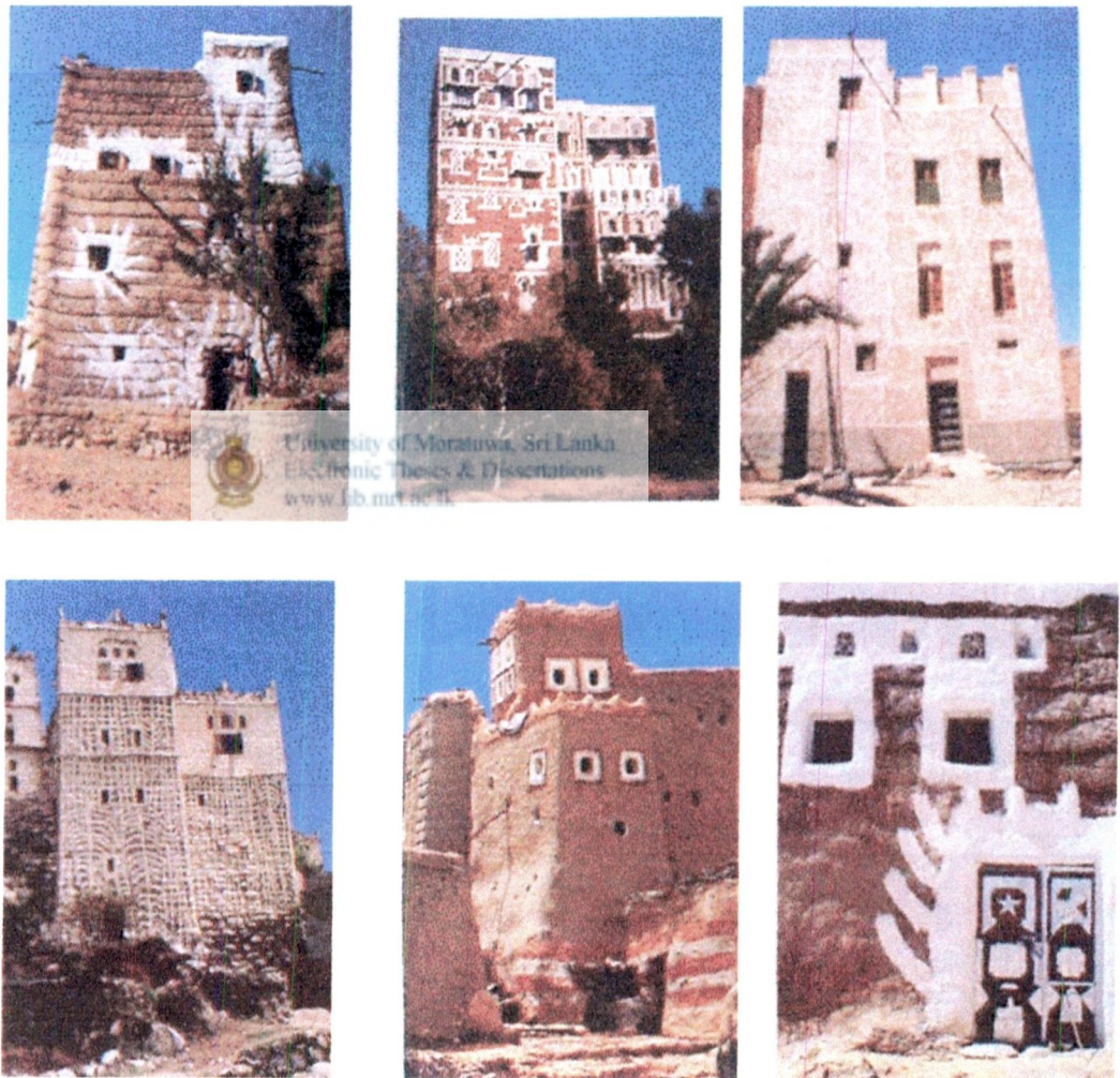
Figure3.6: sample façade survey
