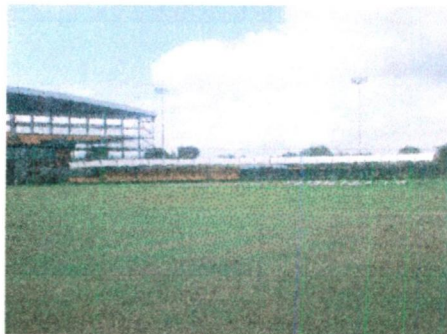
Figure3. : lighting poles almost invisible with the view
