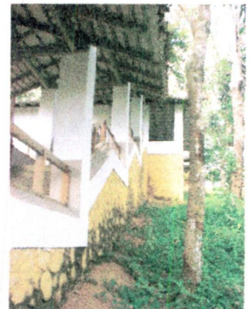
Figure3. :white column showing its presence from the ground with yellow base
