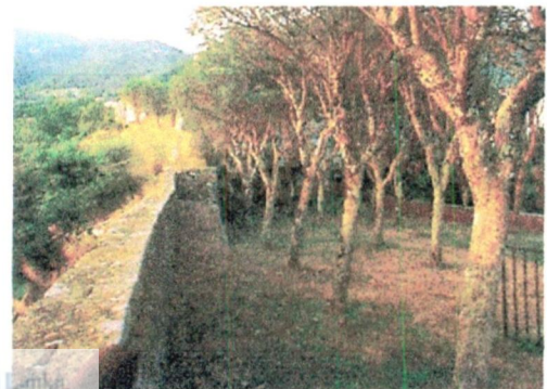
Figure 1.23: demarcated boundary Source: The Most Beautiful Villages of Tuscany
